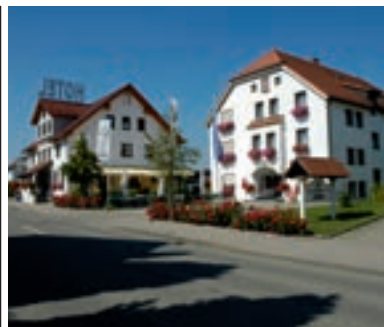
18 Hotel-Restaurant Adler, Westhausen
